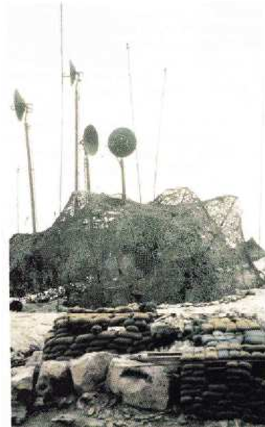
Figure 3.18: Microwave Communications Relay Sites Providing Communications Link Between XVIII Airborne Corps and Rear Area[214]
