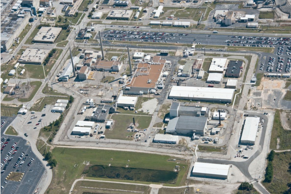
Savannah River Site, 2012
