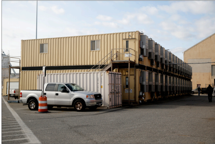
Double-stacked temporary office facilities at Norfolk Naval Shipyard, 2016 (GAO, 2017).
